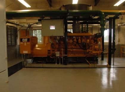
During the fall and winter of 2003, these engines were retired and removed from the building. Building modifications began for the installation of a new 2250 Kw Caterpillar 3516 V16 Diesel Generator. This generator was put into service in June of 2004. This unit is in service today along with the hydro generator that was installed in 1929.
