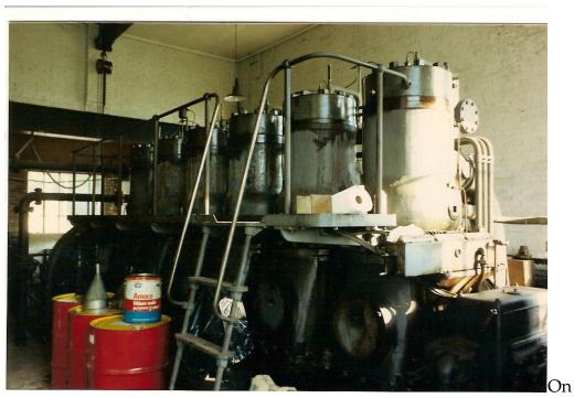
November 1, 1946, the Village Council entered into a contract with Fairbanks Morse to provide one 300 Kw diesel 6 cylinder engine and generator for \$43,200. This engine was installed in March 1948.
