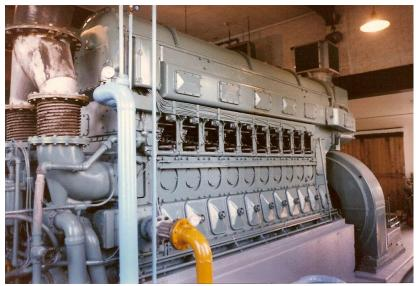
The second of these engines was installed in 1989 making the total capacity of the plant 2.2 megawatts. These engines were built in the 1940's as power for ships and submarines for the Navy during WWII. They served us very well up to turn on the century, when plans began for their retirement due to the need for overhaul and need for more efficient and environmentally friendly equipment.
